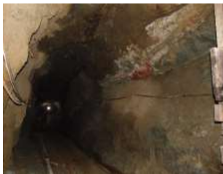
Figure: (8 c and d) Shear plane and breccia zone of underground adit in Nansamsar mine (2)
